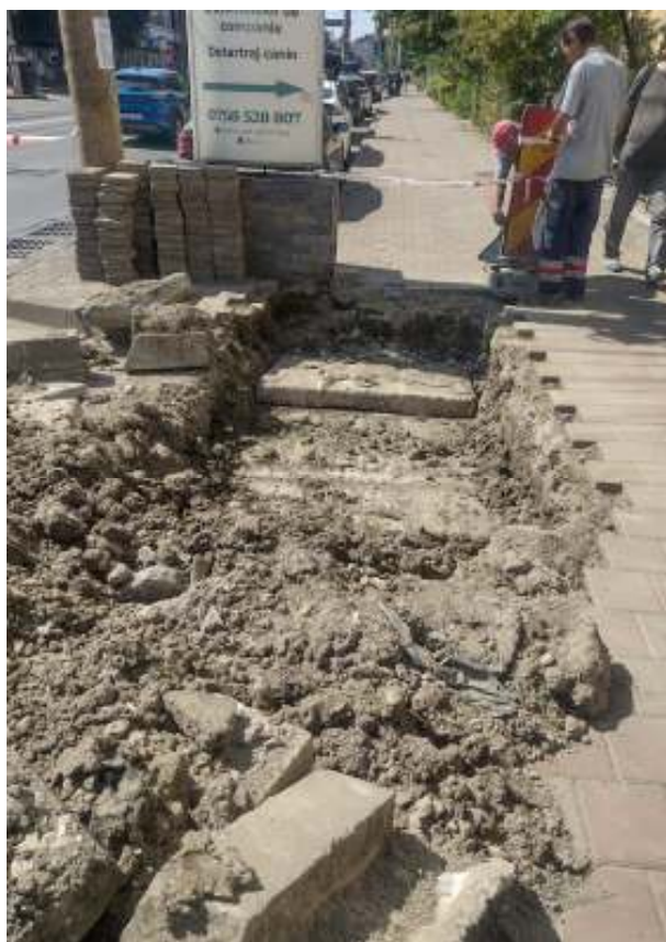
img 10, img 11 Rețea transport magistrala 5 racord Canta 1
